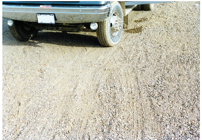
Figure 1. Free-draining, unstabilized subbase with enough fines to be stable during construction but still provide permeability of about 200 ft/day (60 m/day) in laboratory tests. Note that the truck tires are not causing excessive rutting or displacement of the subbase material.
