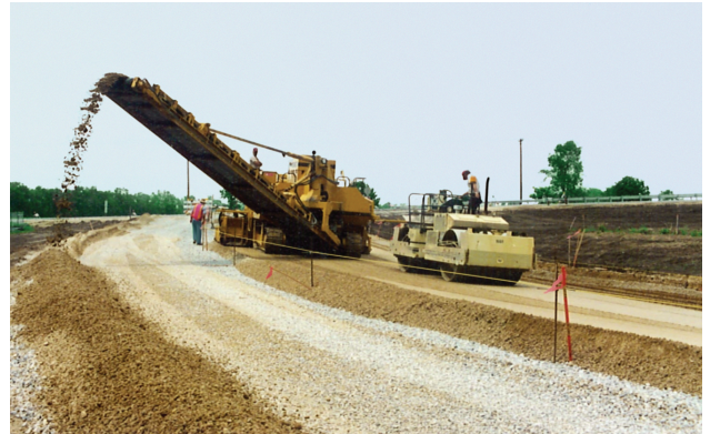
Figure 1. Grading of an unstabilized subbase.
