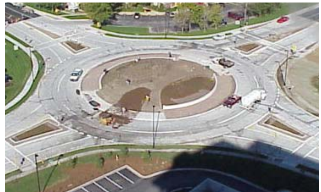
Figure 5. Completed concrete roundabout.
