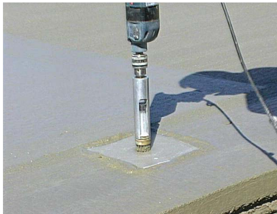
Figure 4. Obtaining concrete sample for Air Void Analyzer.
