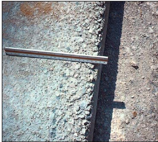
Figure 5. Edge erosion of freshly-placed slab due to rain.
