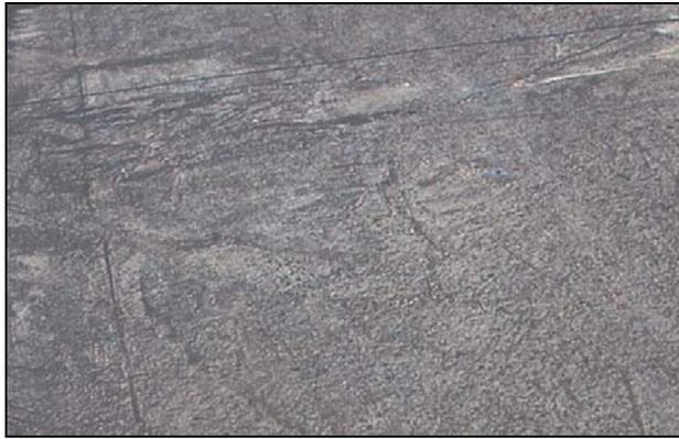
Figure 1. Marring of the pavement surface due to plastic sheeting. Does not require remediation unless ride quality or skid resistance is unduly affected.
