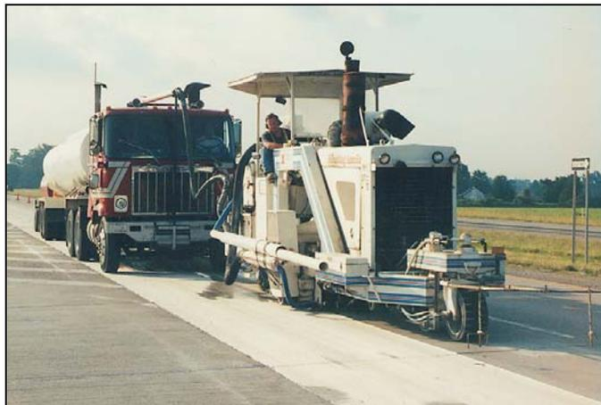
Figure 4. A diamond grinding machine is used for removing the non-durable surface, re-texturing the pavement, and smoothing out the ride.
