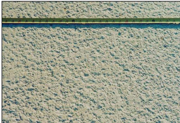
Figure 2. Typical scaling of concrete pavement due to non-durable paste on surface.
