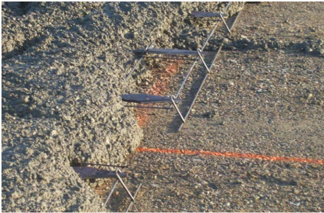
Figure 7b. Double taper plate basket [photo courtesy of Greenstreak Group, Inc.].
