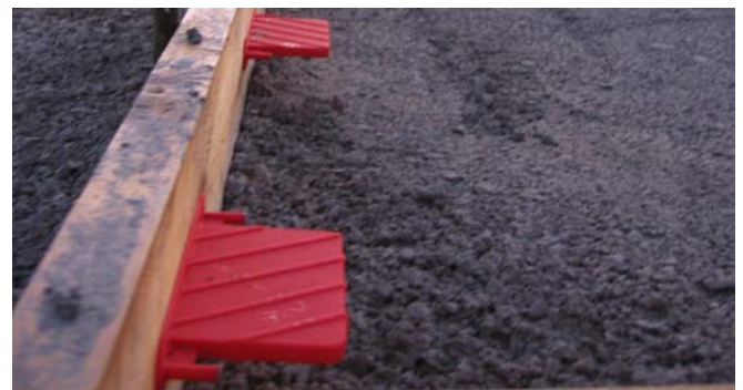
Figure 6b. Square pocket former for rectangular plate dowels installed on a wooden construction joint form [photo courtesy of Greenstreak Group, Inc.].
