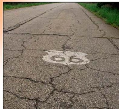
**Surface Cracking:** Degradation resulting from cycles of heating and cooling; Such cracking causes a rough ride.
