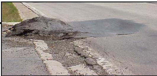
**Shoving:** Caused by heavy traffic stopping and starting on the thin pavement layers common in pavements that don't use concrete; this deformation can cause substantial damage to vehicles.
