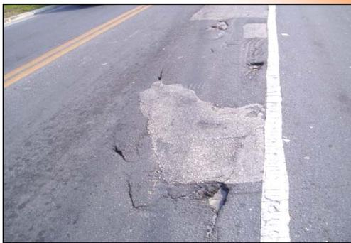
**Potholes:** Degradation caused by a combination of the freeze-thaw cycling and traffic. Potholes may cause extreme damage to vehicle suspension and are costly to repair.
