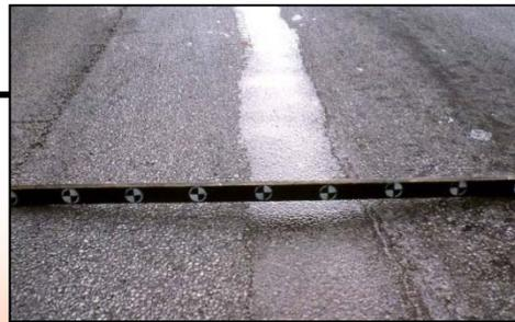
**Rutting:** Deformation under the wheel paths in pavements that don't use concrete. Water-filled ruts can cause vehicles to hydroplane at high speeds.
