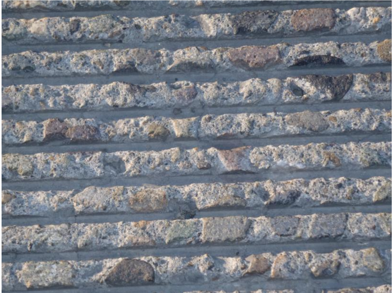
Figure 23 Apparent Attrition of NGCS Surface from Studded Tire Damage
